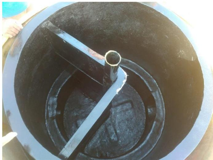
Fig; 5 constroction of Digester
